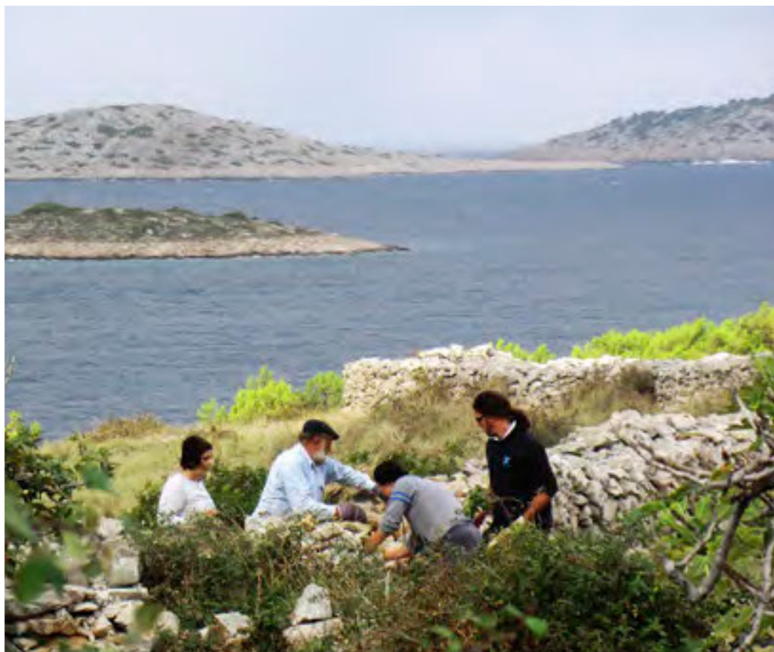
Kornati: Building and renewal of dry-stone walls, 2015. Photo by Vilma Stopfer, © Association 4 grada Dragodid.
